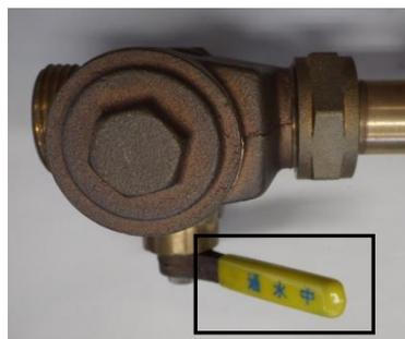
『閉栓中』 (closed) is shown on the lever.
